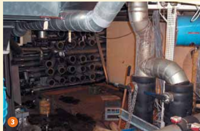
The old AHU is removed
