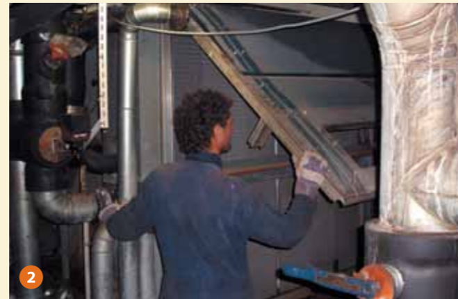
Dismounting of the old AHU
