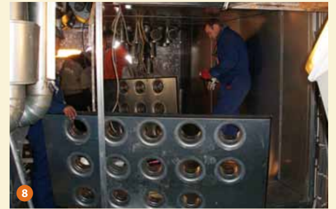
Installation of the spiro pipes connection to the AHU.
