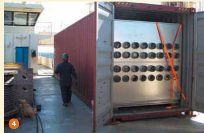
This time the AHU was delivered complete, ready for easy dismantling and rebuilding on site.
