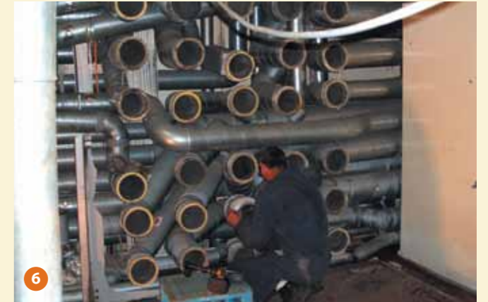
The spiro pipes may be slightly adjusted
