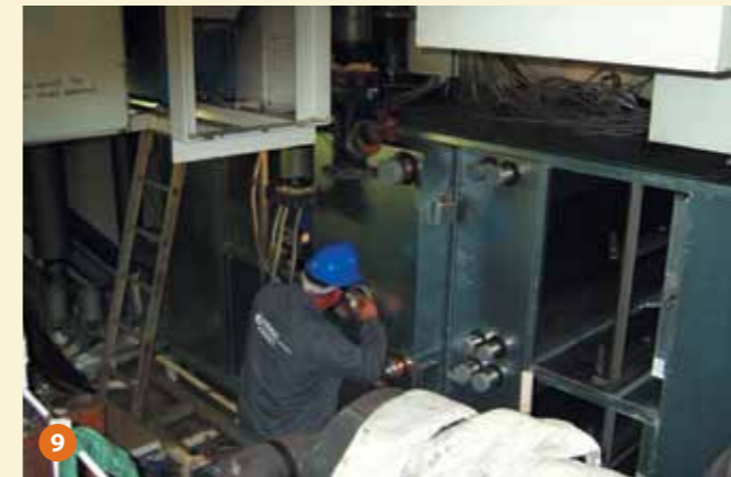
The new AHU is under installation
