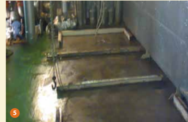
The base frame for the new AHU is installed
